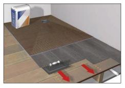
Where the first waterproof board will sit, spread the board fixing adhesive onto the floor and drag the notched adhesive trowel across the surface. The notched adhesive trowel will make a ribbed pattern which will leave just the right amount of adhesive on the floor.
