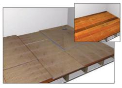
Measure the entire floor area and plan the layout on a sheet of paper. Decide if any of the waterproof boards need to be cut and if they do, cut them now using a hard point saw. Lay the entire pack out across the floor area to check the fit.
