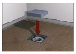
Step 26 Place the disposable tiling aid into the shower drain hole on the shower tray. The tiling aid provides the edge that needs to be tiled up to whilst protecting the drain from debris.
