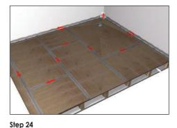
Apply a thin layer of tape sealer to one edge of the floor and adjoining wall approximately 60mm wide on each.
